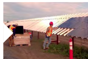
Panels installed on racking
