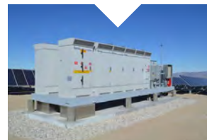
Inverter/Transformer Skid
