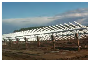
Racking mounted on piles
